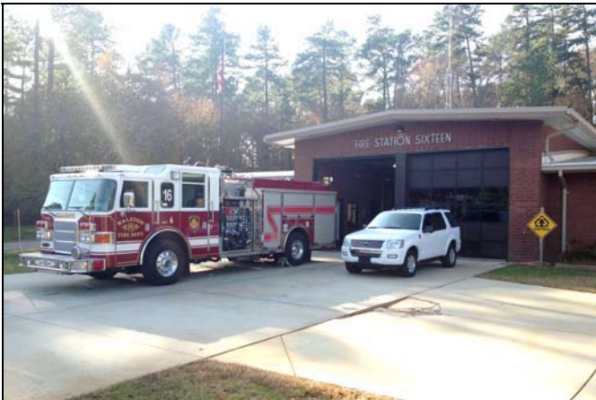
On Nov. 29, the platoon Deputy Fire Marshal (Car 40) was moved to Station 16. The unit was relocated from Station 21 in preparation for relocating Rescue 1.
