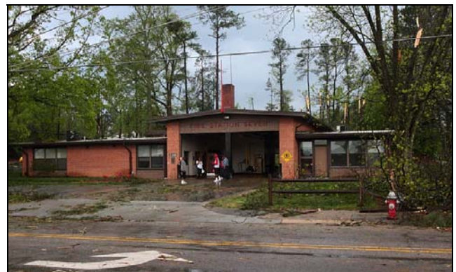
Fire Station 7 on Glascock Street
